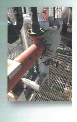
With our custom design process we can create removable insulation covers to satisfy virtually any application, and with the highest quality materials we will ensure excellent performance and long life. All covers include an aluminum tag engraved per customer spec (i.e. Valve #) in case replacement is required.
