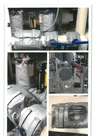
We manufacture custom-fitted, removable and reusable thermal insulation covers for commercial and industrial mechanical piping and equipment. Removable pads reduce energy costs and maintain process temperatures while protecting personnel and equipment from hazards. Easy to install and remove.
